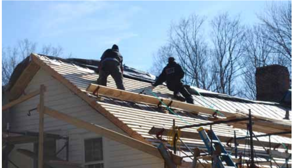
Installation of the breathing grid on the 1820s ell
