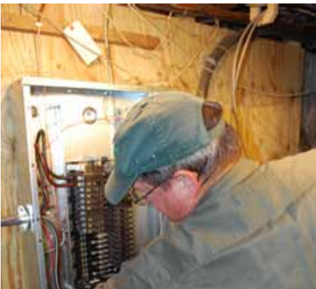
Installation of the new electrical panel
