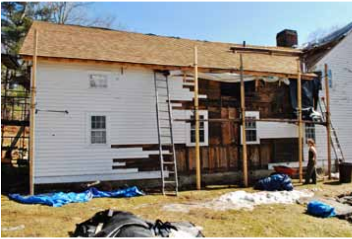
Exposed west wall of the 1820s ell, with completed roof
