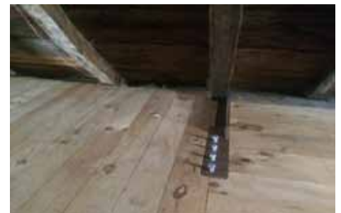
Steel joint support in the attic
