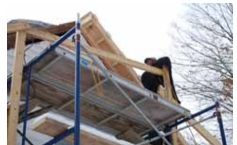
Replacement of roof overhangs on ell
