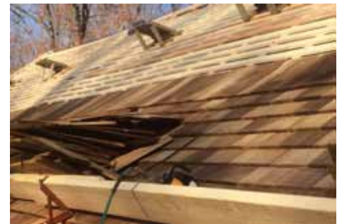
New cedar shingles on the front roof
