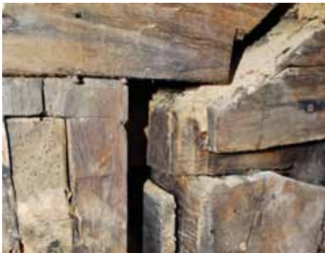
Juncture between 1760s and 1820s frames
