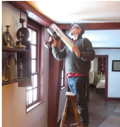
Probing the beams for soundness
