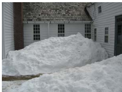
5-foot snow piles below the salt box roof
