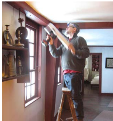
Probing the beams for soundness
