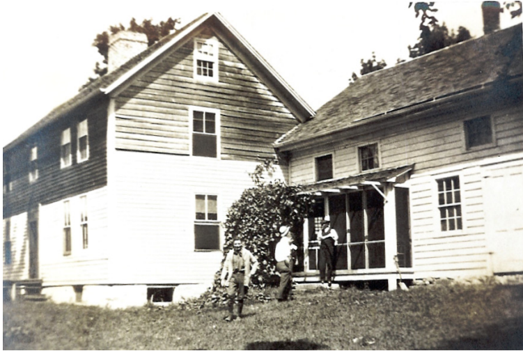
Ca. 1900, the Carrington family owned the house and farmed the land. Note the two-toned clapboards, gable overhangs and enclosed porch
